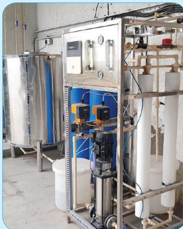
4000 LPD 6 stage Drinking water plant for Amazon Campus, Hyderabad
