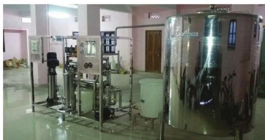
144 KLD RO Plant for Super PS Plant
